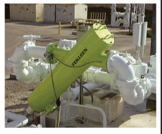
that the new filter operate on a small amount of electricity. When the Watsonville, Calif. Wastewater Treatment Facility's 20-year-old filter needed replacing last year, one major concern was the conservation of electricity.
